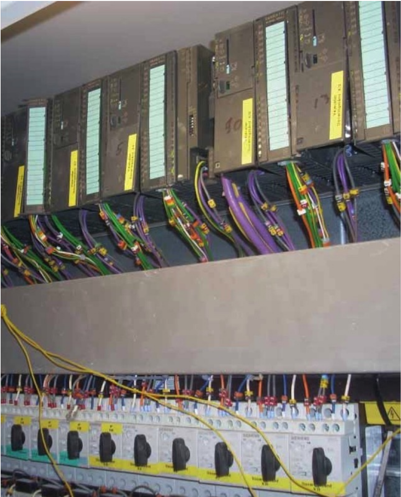
Fig. 2: Siwarex FTC weighing modules during commissioning they provide fast, continuous monitoring and control delivered directly to Nopa's control room.
