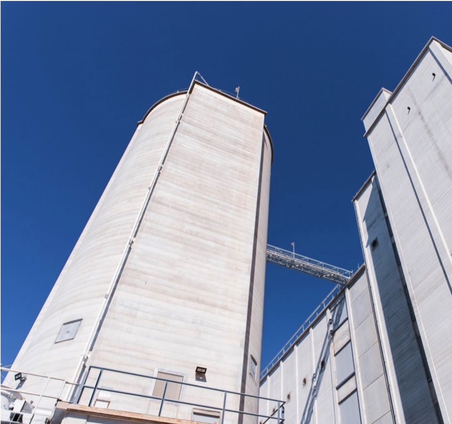
Ardent Mills new Port Redwing facility in Gibsonton, Florida, stands tall among the world's mills.
