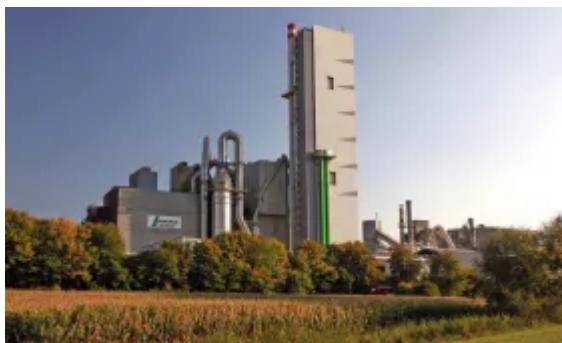
Fig. 1: In the course of a modernisation project at Lafarge's Wössingen cement plant, the capacity of the bucket elevator to the mill bunker has been increased considerably. (Pictures: ©Beumer Group)
