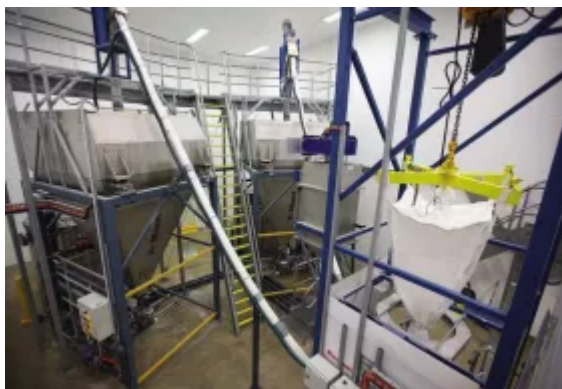
Fig. 1: Recently, Prominent Fluid Controls has supplied equipment for large water-fluoridation plants; the major pieces of equipment are a bulk bag discharger, a dust containment system, and a flexible screw conveyor. (Pictures: ©Flexicon (Europe) Ltd.)
