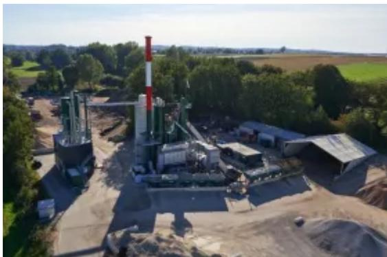
In the Aichach asphalt mixing plant, wood dust is used as a fuel instead of heating oil by the Benninghoven EVO Jet multi-fuel burner. (Pictures: ©Wirtgen Group)
