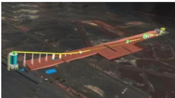
The F'Derick project in Mauritania. From right to left, the primary and secondary crushing stations, leading to the transfer tower and train loading station via a network of conveyor installations. This complex system is the result of our expertise in delivering complex bulk material handling systems. (Picture: ©TAKRAF GmbH)
