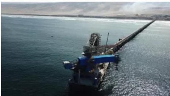
The copper ore is transported from the mainland to the ship loader via a conveyor system. (BEUMER Group GmbH & Co. KG)
