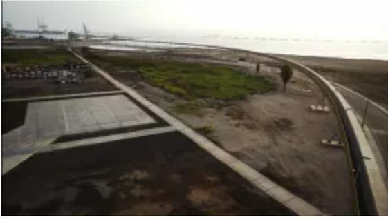
The pipe conveyor passes through the port: This is the final curved section before the transshipment tower for transfer to the port terminal.
