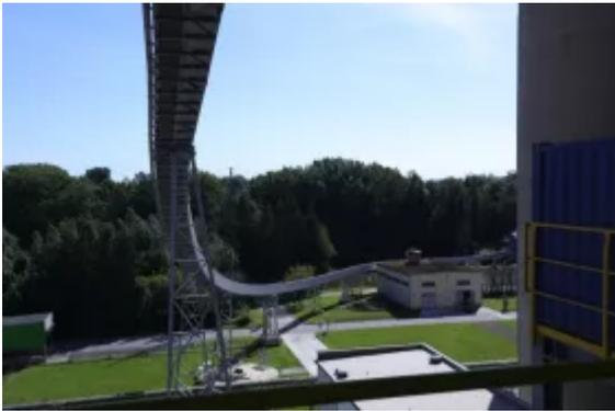
The U-shape conveyor is able to cope with tighter curves than a troughed conveyor and transport larger mass flows than a pipe conveyor.
